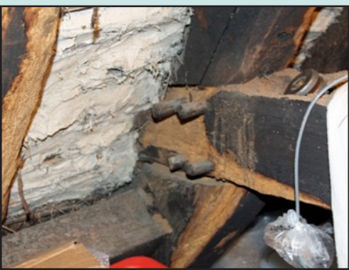
TOP LEFT: Cruck visible on the landing of Studley Grange farmhouse. © Wiltshire Buildings Record.
